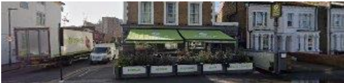
Front elevation facing West
